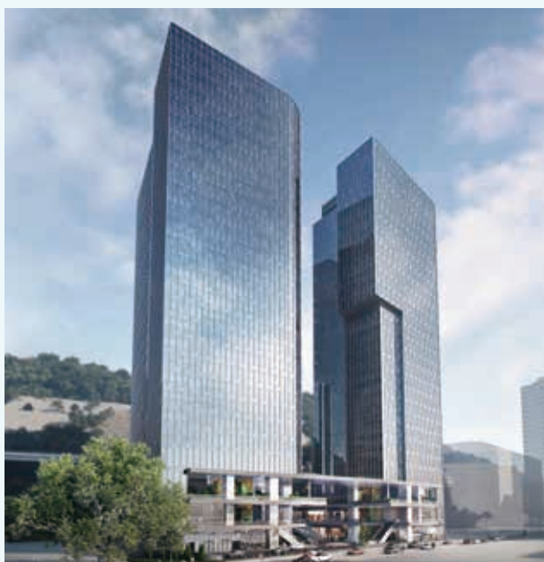
Front view of PORTAS
